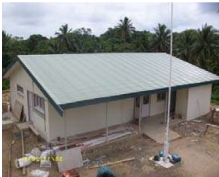
Figure 2. Loma Nursing Station that was relocated to higher
