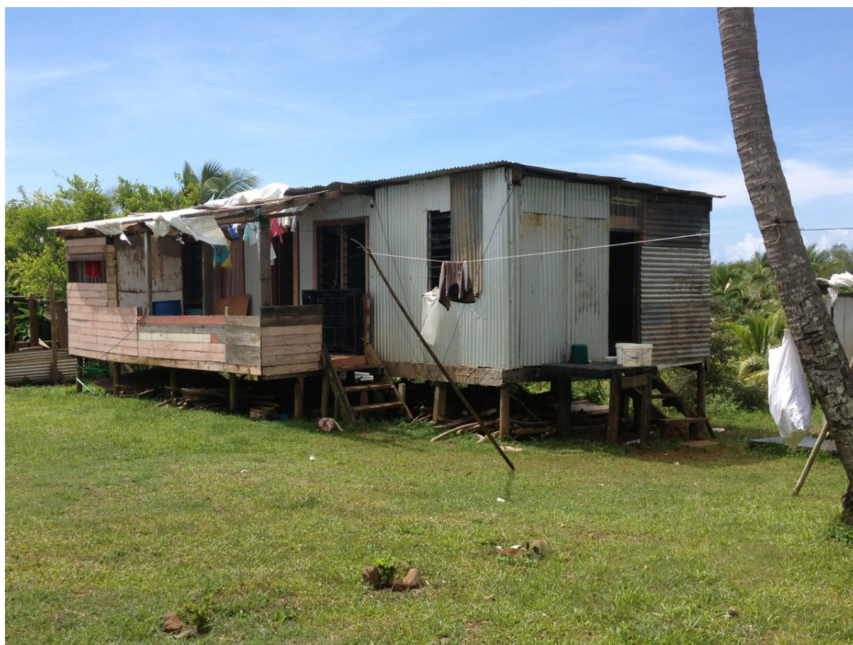
iTaukei house in the Ba River catchment. Note that the house sits on stilts due to previous exposure to flooding.
